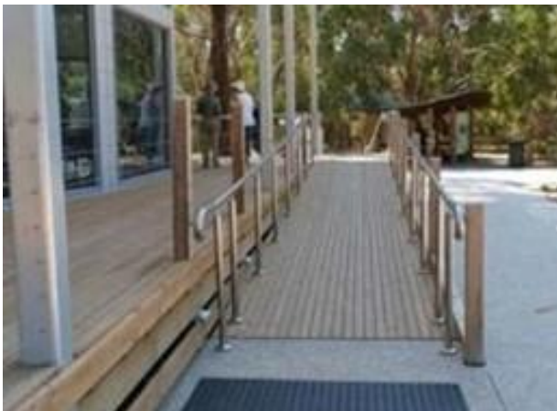
Ramp access to the Visitor Centre
